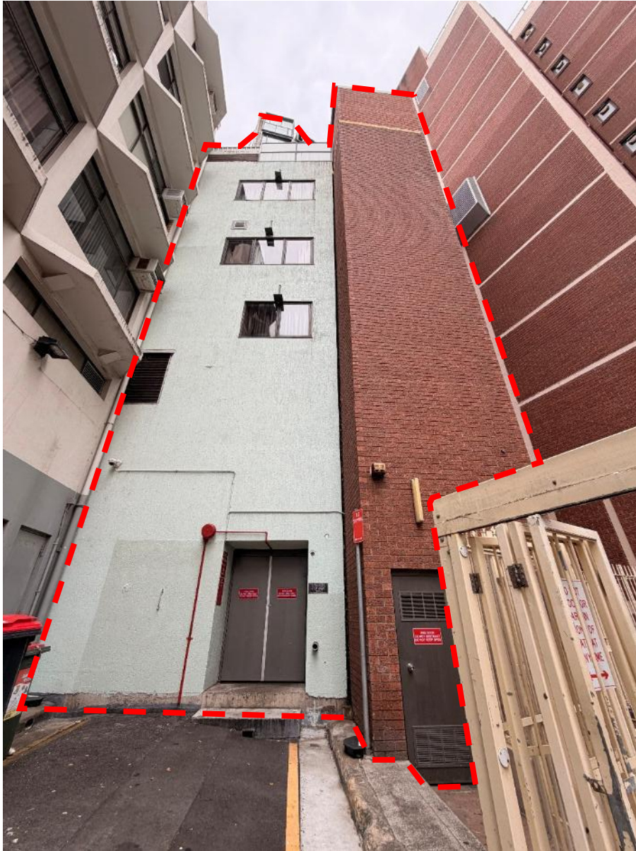
Figure 5: Rear of the site (dashed red) viewed from Earl Street, looking south
