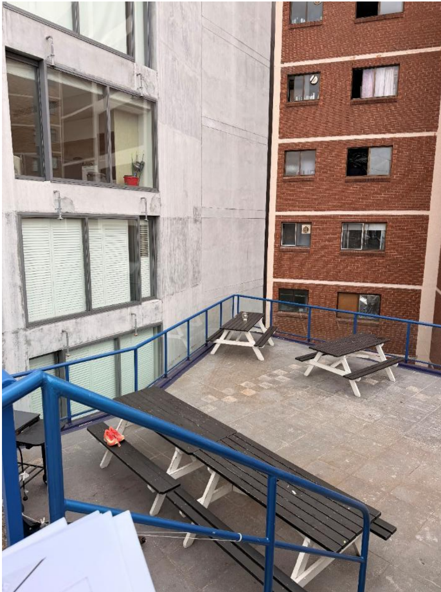
Figure 11: Western side of existing rooftop terrace at the front of the building looking west
